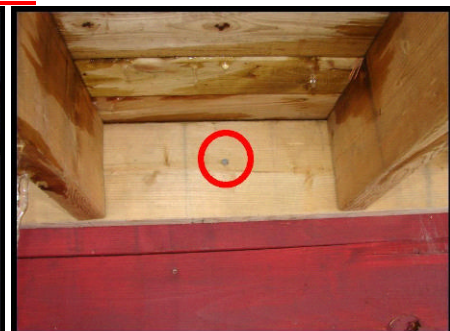
Deck nailed to structure.
